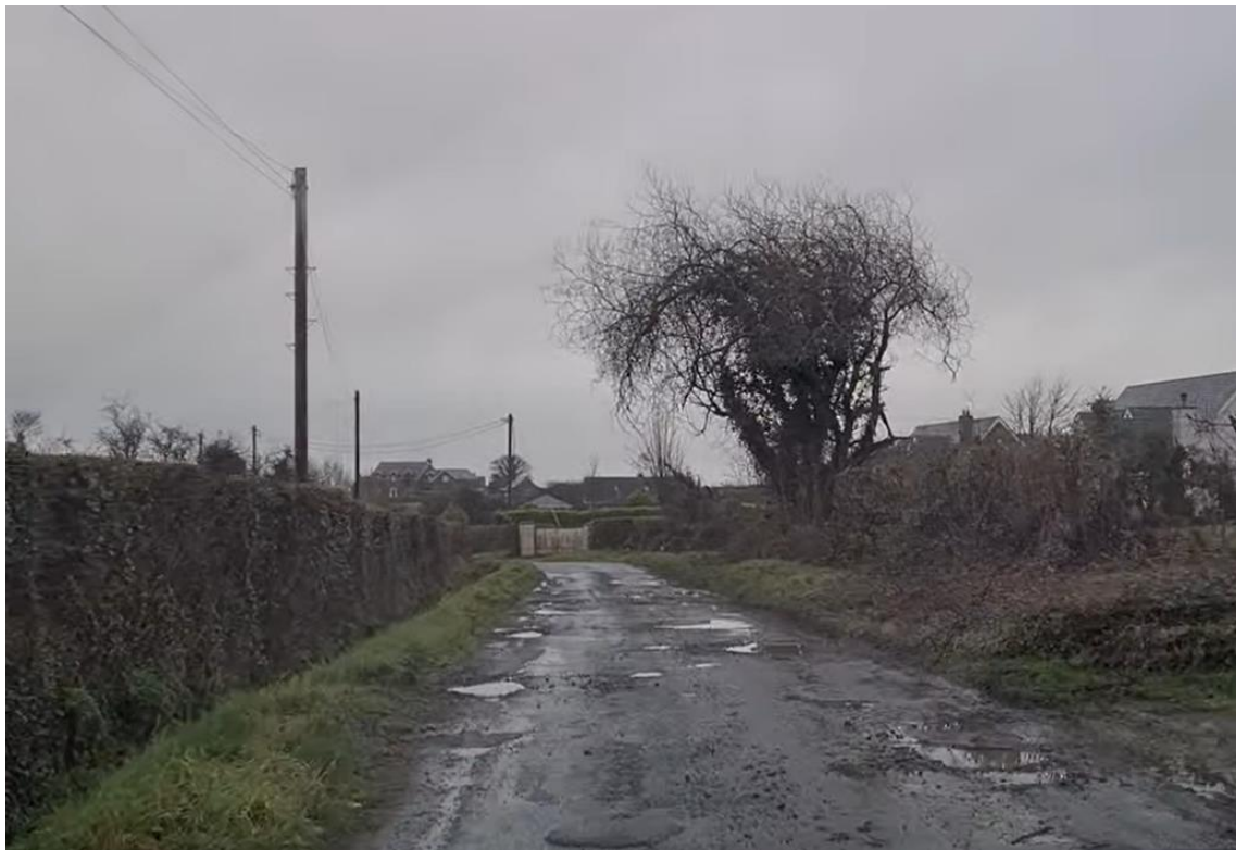
Existing LT63121-1 Road Surface
