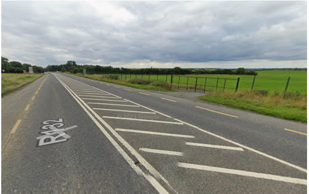
Existing R132 Road Carriageway including a Solid Hatched Median (Google Image)
