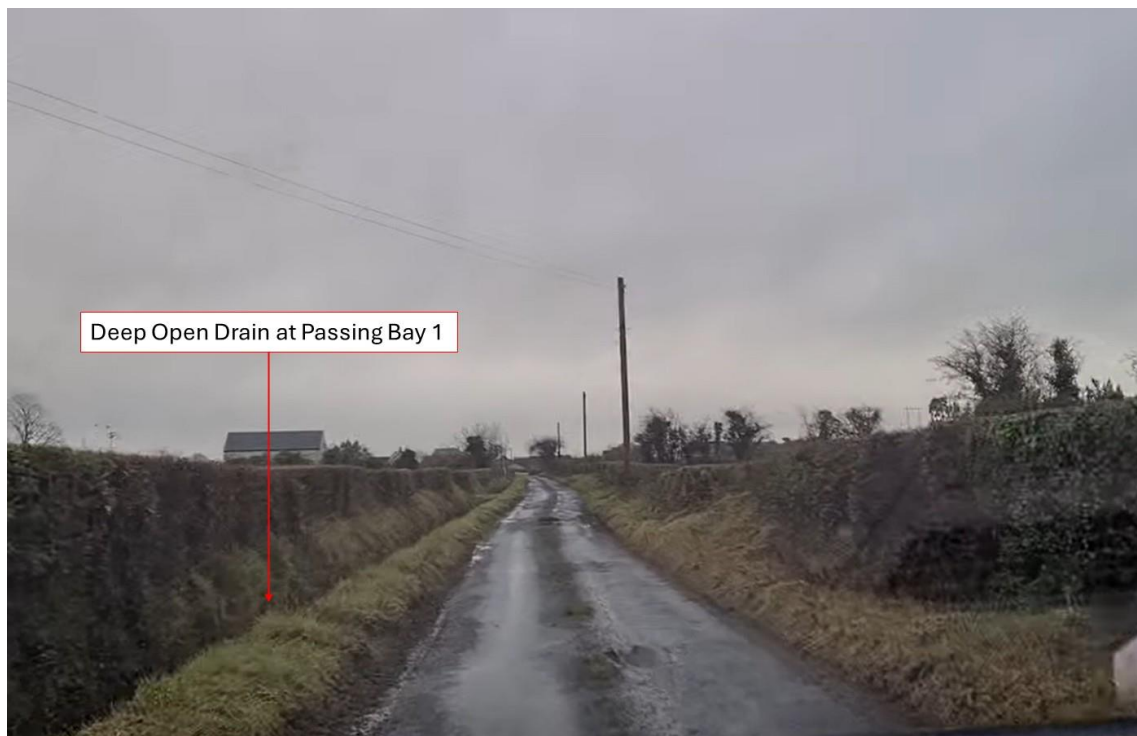
Existing Open Drain and Ditch at Passing Bay Location 1
